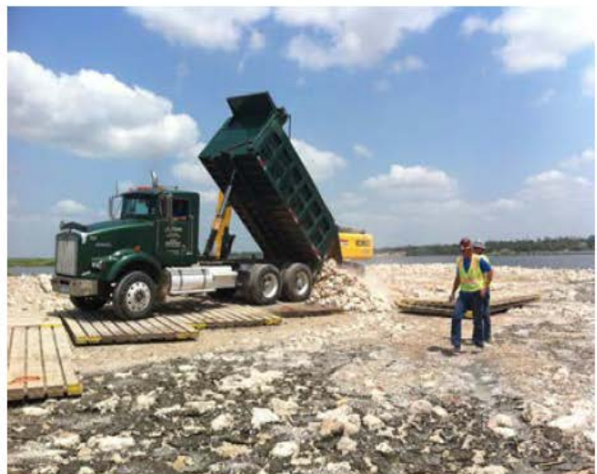
Dump truck off loading rock for placement
